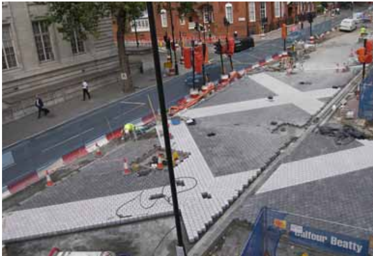
Exhibition Road works in progress
